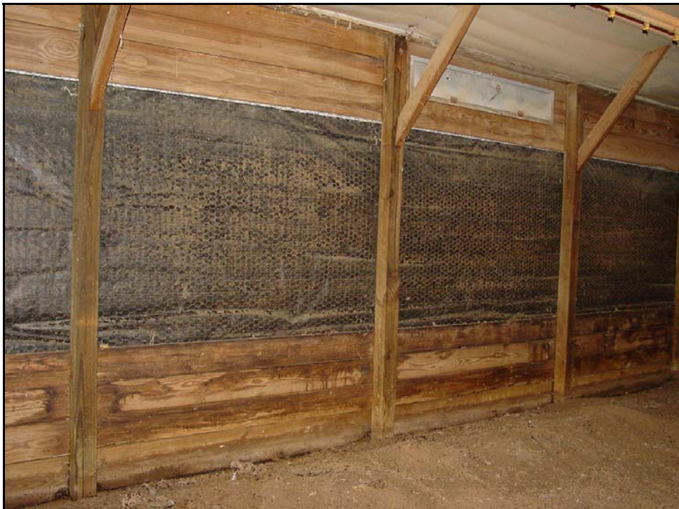
Interior Curtain Wall Prior To Treatment – October 2005
