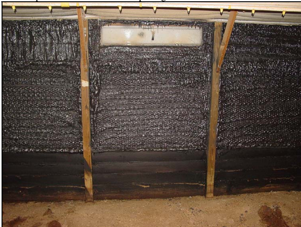
Completed AG-Tite Curtain Opening And Sidewall – October 2005
