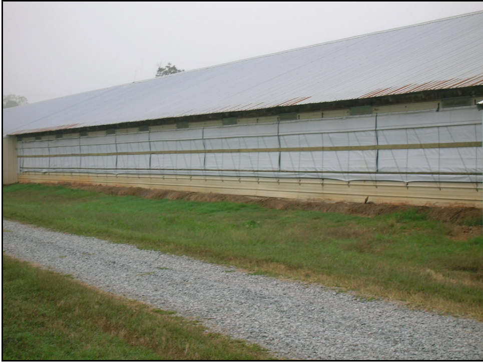
Exterior Curtain Nailed Down With Treated 1" X 4" Boards – October 2005
