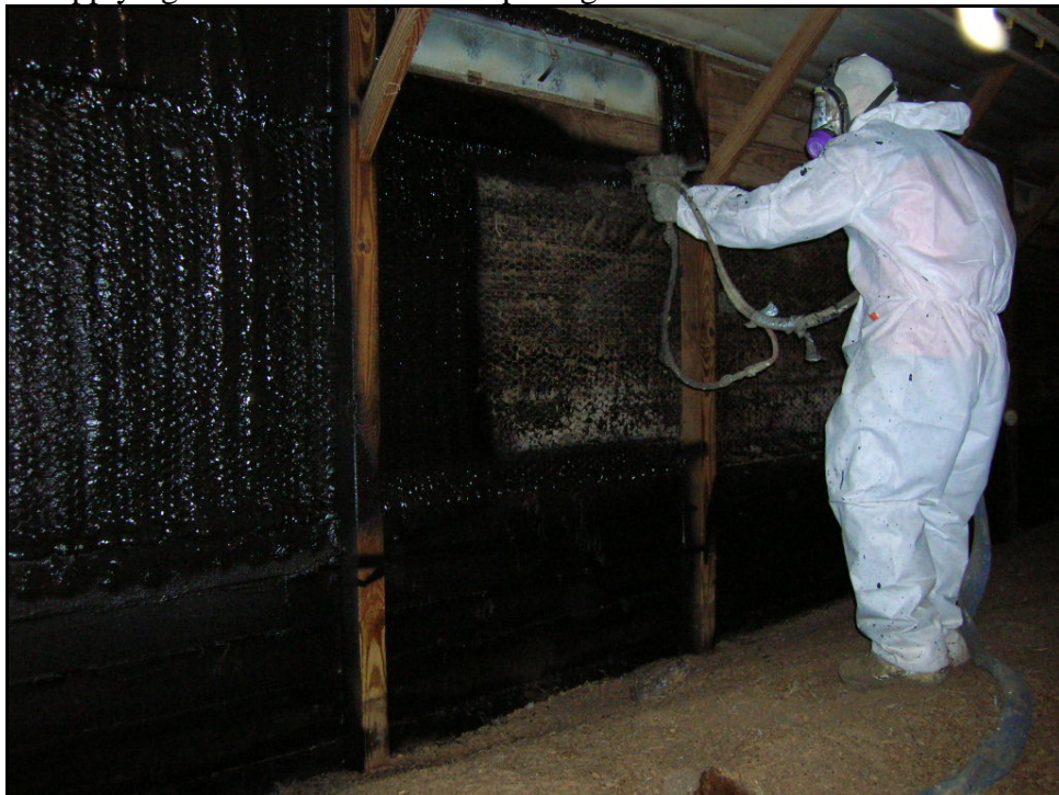
Applying AG-Tite To Curtain Opening And Sidewall – October 2005
