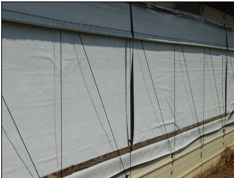
Exterior Curtain Wall Prior To Treatment – October 2005
