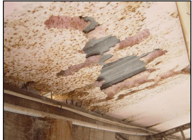
Figure 3. Mice taking advantage of beetle damaged insulation.
