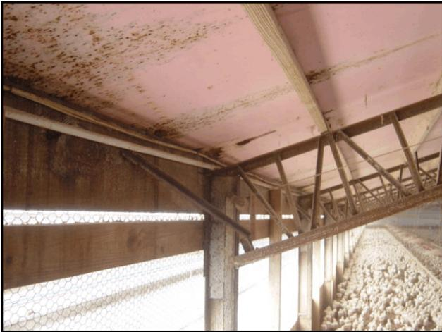
Figure 2. Beetle damaged ceiling insulation.
