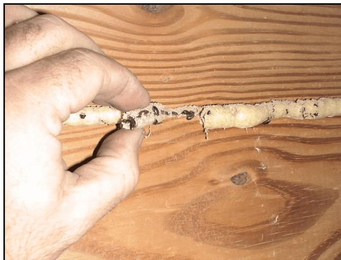
Beetle damage to "foamed" crack.
