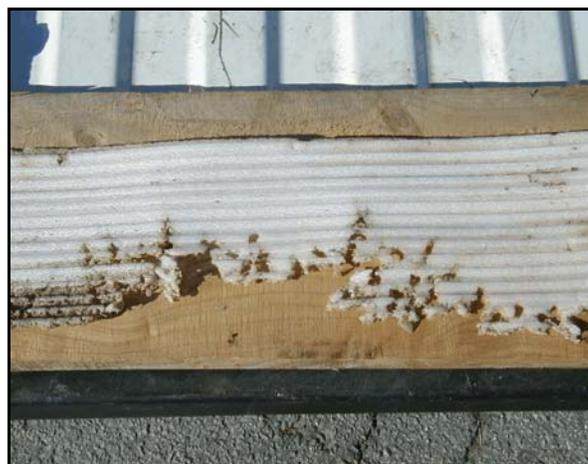
Figure 6. Beetle damaged sill sealer.
