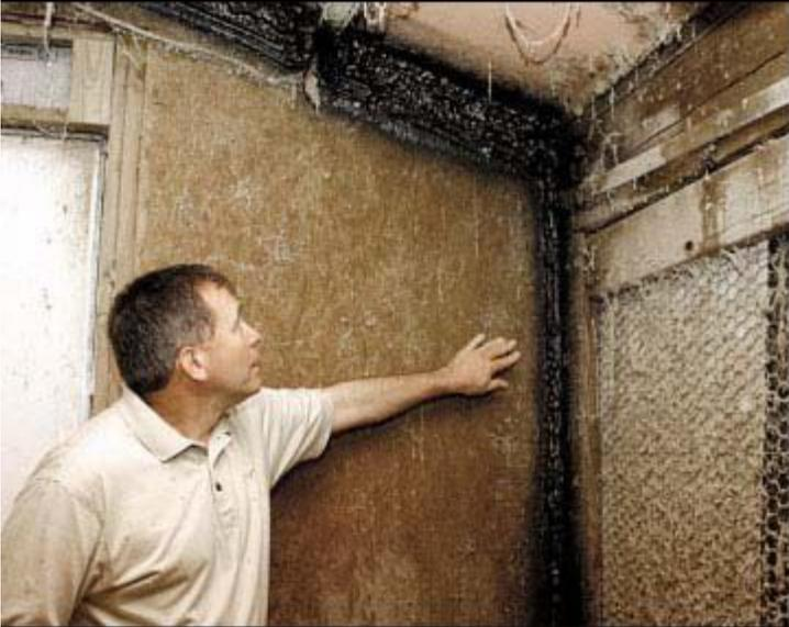
Bill Collins, the general manager of Lincoln-based Ag-Tite, shows how his company's sealant fills gaps and prevents air loss from the joints in chicken houses. The dark areas are where the sealant has been applied.
